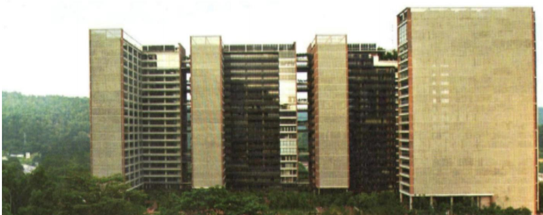
Figure 5.2.2: Building façade where wind tunnel effect occurs at PJ Trade Centre
