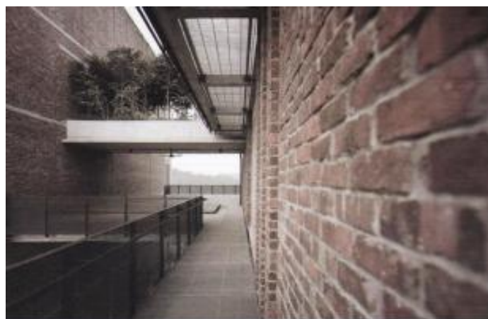
Figure 3.2.1.3: Exposed area with brick walls made of red mud over-burnt bricks at PJ Trade Centre
