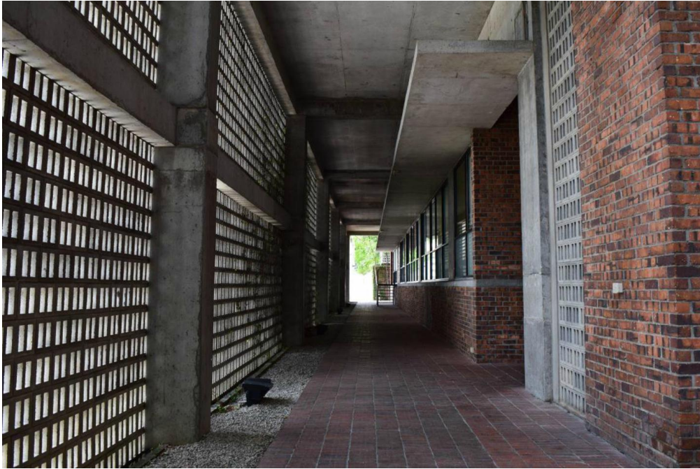
Figure 3.2.2.3: Concrete vent block façade acting as double skin and use of concrete vent block wall on the interior.
